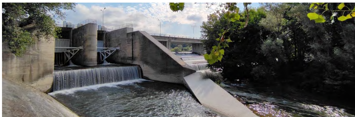
TOXOTES DAM – VIEW FROM DOWNSTREAM, RIGHT BANK
