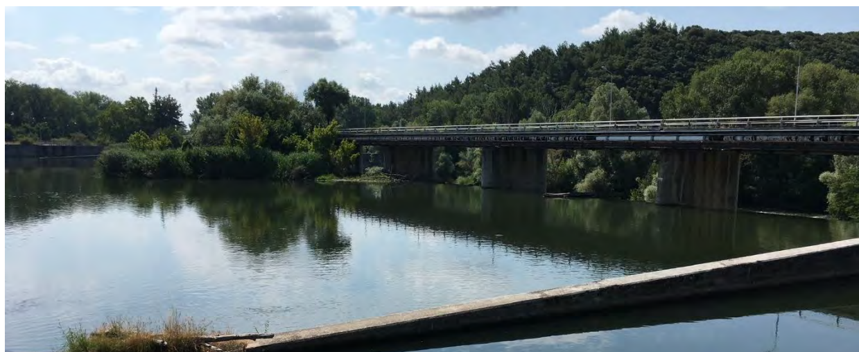
TOXOTES DAM – VIEW FROM UPSTREAM, RIGHT BANK
