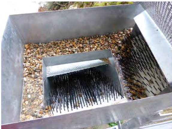
REST POOL FILLED WITH GRAVEL (LEFT) AND STEEL SHEET CHANNEL (RIGHT)
